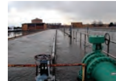
Treatment tanks overflowed at Hunts Point, Bronx WPCP March 2001 storm; unusually high tide elevations prevented discharge of treated sewage into East River, caused back-up
